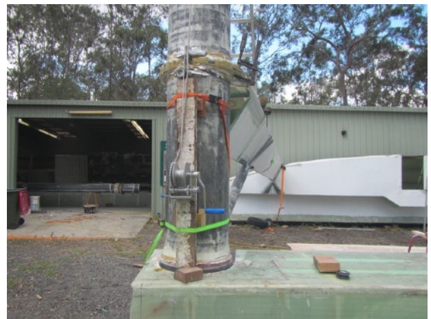
5 to 1 winch on bottom
