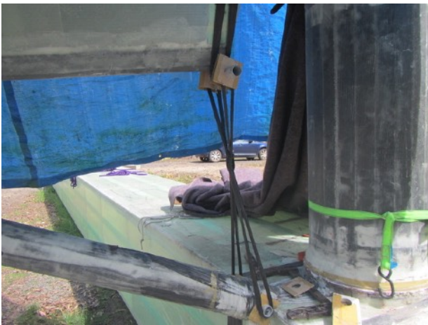
Beam to hull bracing 1
