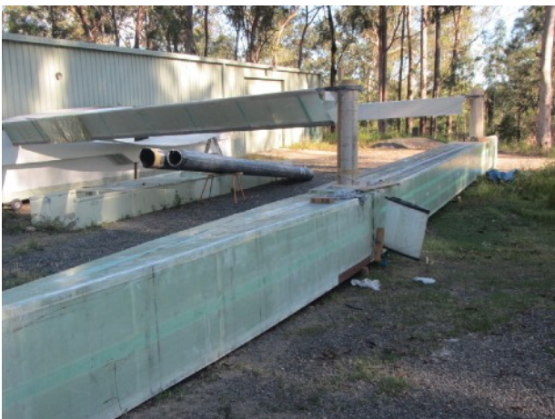
2nd beam fitted
