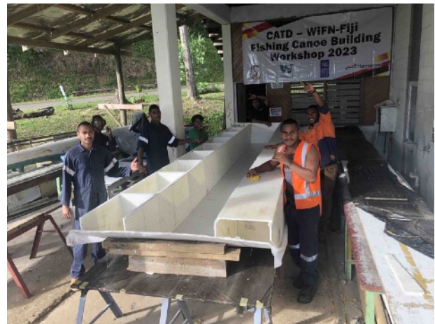
Water taxi build
