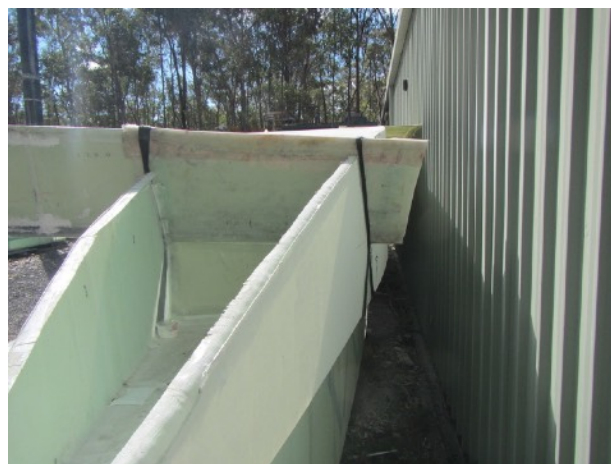
Ready for fore deck
