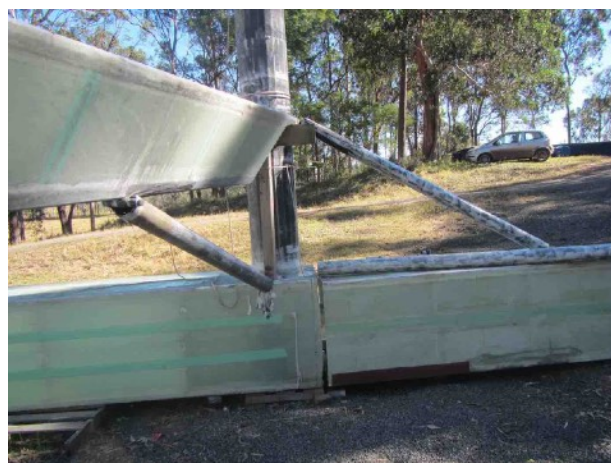
Carbon struts supporting the beam and mast
