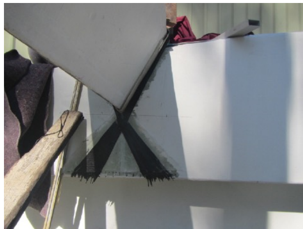
Beam socket reinforcing
