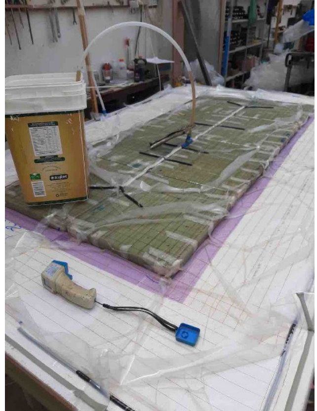
Beam bulkheads infused
